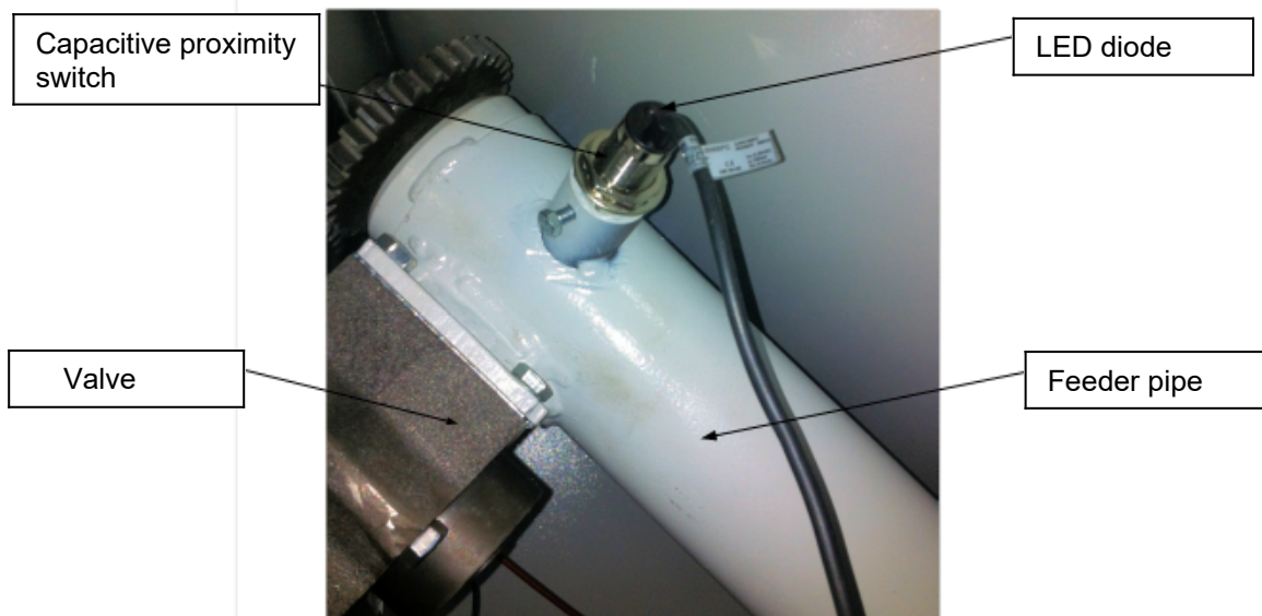
Figure No. 16 Location of capacitive proximity switch
